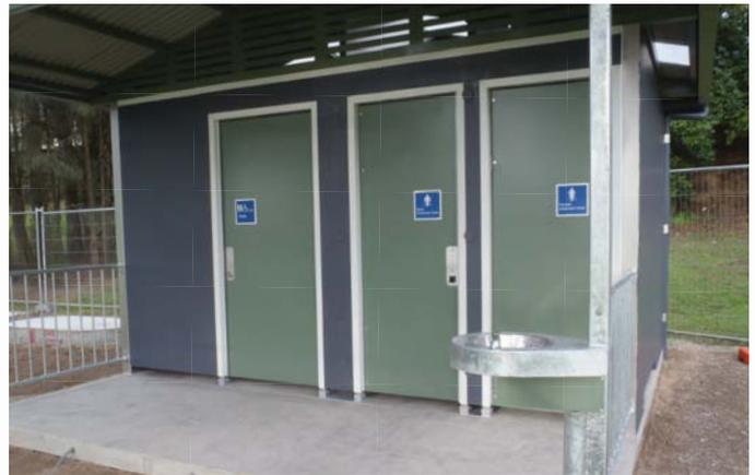
Our standard sink column ntegrated as the sink column housing all plumbing and hot-dipped galvanised as a finished fabricated element.
